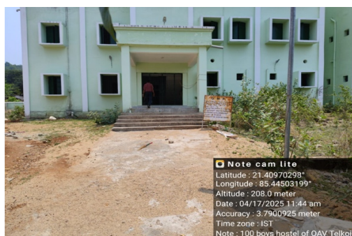
Picture 7 : Locked Hostel under OAV, Telkoi
