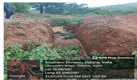
Photograph 1: Sheet rock encountered during execution of UGPL Bisamagiri.
