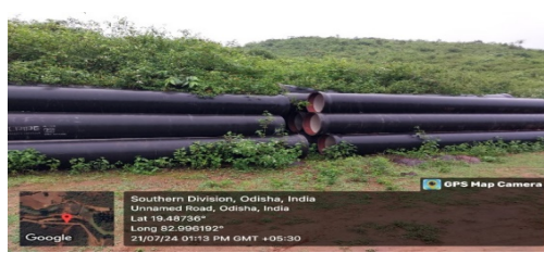
Photograph 5: Stacking of UGPL pipes for Bisamgiri MIP, Bhawanipatana
