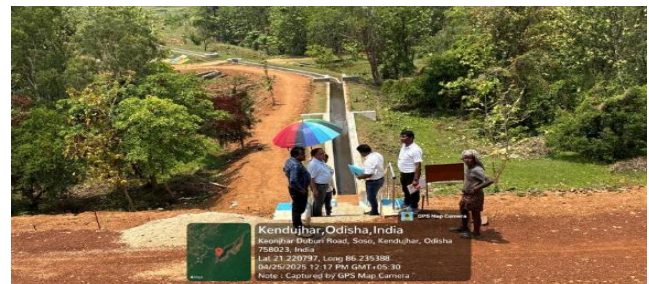
Photograph 6: Canal lining works in Bahiya MIP, Anandapur, Keonjhar
