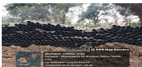
Photograph 4: Stacking of UGPL pipes for Bhatpur MIP, Rayagada
