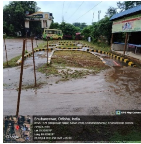
Picture-7: Waterlogged, uneven testing track at Bhubaneswar
