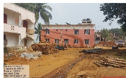
Picture 8: Damaged infrastructure in Satpada
