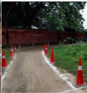
Picture-12: Uneven testing track at Cuttack
