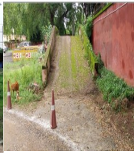
Picture-13: Unusable gradient at the testing track at Cuttack
