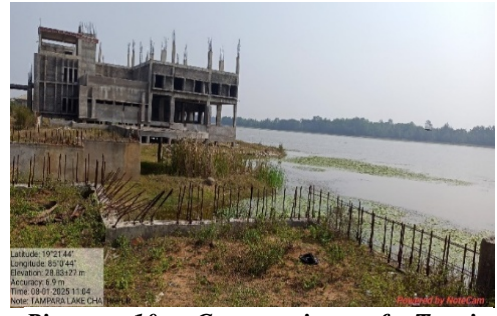
Picture 10: Construction of Tourist Reception Centre Block at Tampara lake under Swadesh Scheme
