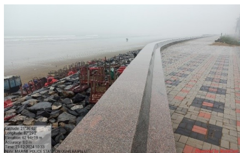
Picture 7: Service road and stone embankment in Udayapur PRF area
