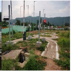
Picture-10: Damaged testing track at Keonjhar
