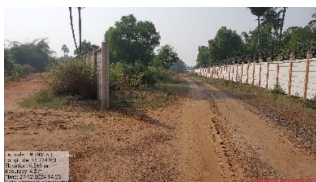
Picture 12 : Boundary walls of STA and Shree Jagannath International Airport
