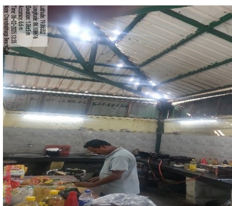
Picture 2: Chandrabhaga Beach Café, Cooking activities in a shed with damaged roof
