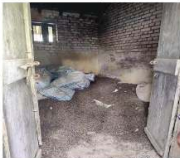
Photograph 3.3: Drugs kept in Muddamaal Room due to absence of dedicated storage facility
