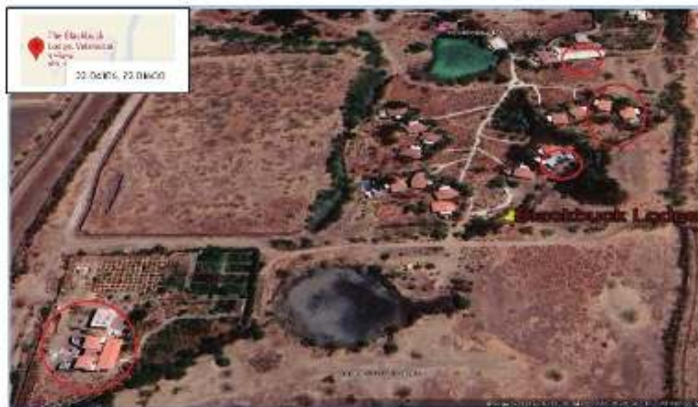
Photograph 3.2: Image of the Lodge as of 11 May 2024 - Construction of additional structures shown within Red circles
