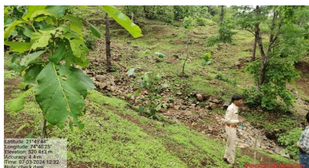
Figure 15: A picture of a Checkdam (soil conservation measure) in Madhya Pradesh
