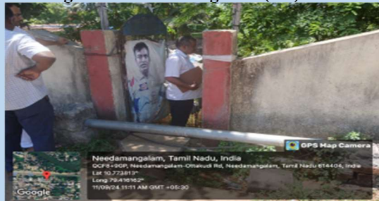
Fig. 2.8: Unauthorised entry from PF to a dwelling unit at Nidamangalam (SR)
