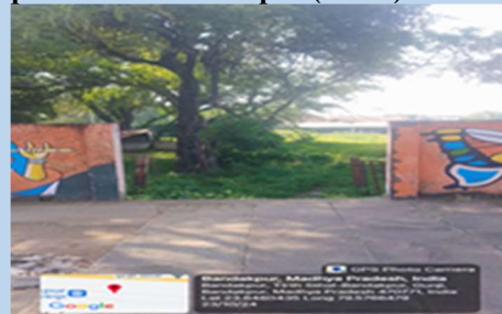
Fig. 2.7: Unauthorised entry to platform at Bandakpur (WCR)
