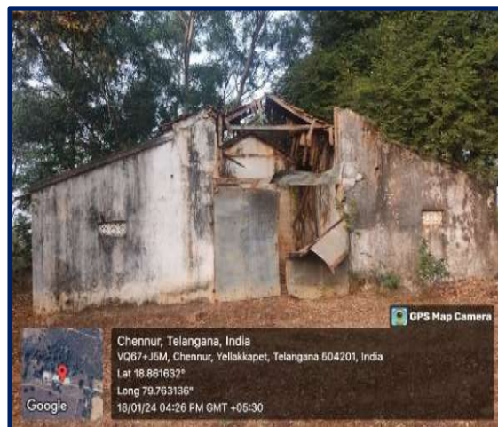
Coordinates - Lat – 18.861632°, Long – 79.763136° Picture 11 - Garage at BSMTC Chinnoor
