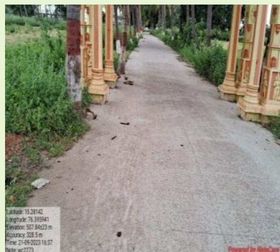
Picture No. 5.11: Non execution of side drainage work in Bhattarahalli Anjaneya Road, Hospete Taluk.
