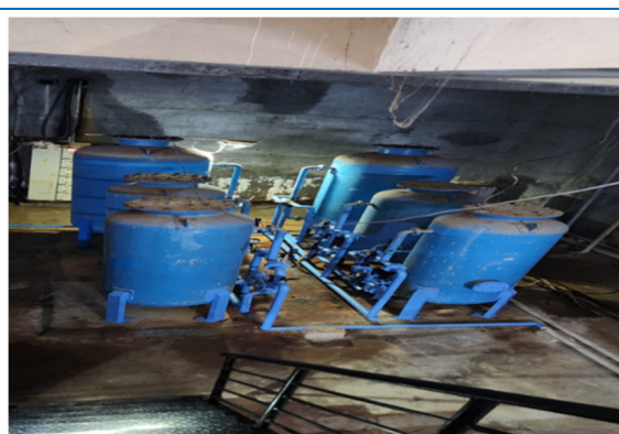
Picture 11.17 Non-functional Water Treatment Plant (Tirupati Campus)
