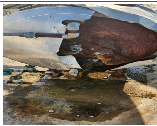
Picture 11.21 Damaged solar water heater (Tirupati Campus)
