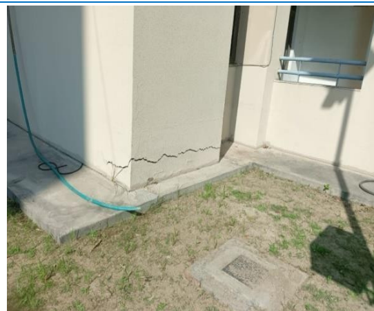
Picture 11.8 Horizontal cracks near base of Staff Quarters (Noida Campus)
