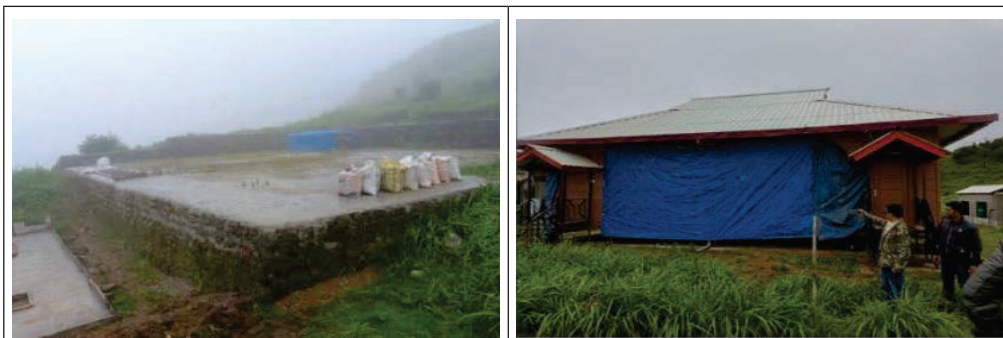
Fig. 3.4: Under construction cottages at Tonglu, Darjeeling
