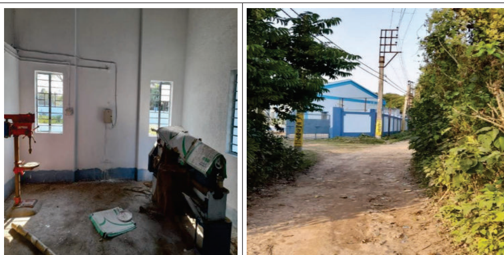
Fig. 4.4: Unutilised machines and earthen narrow approach road in the CFC
