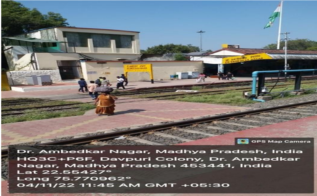
Dr. Ambedkar Nagar Station of Western Railway
