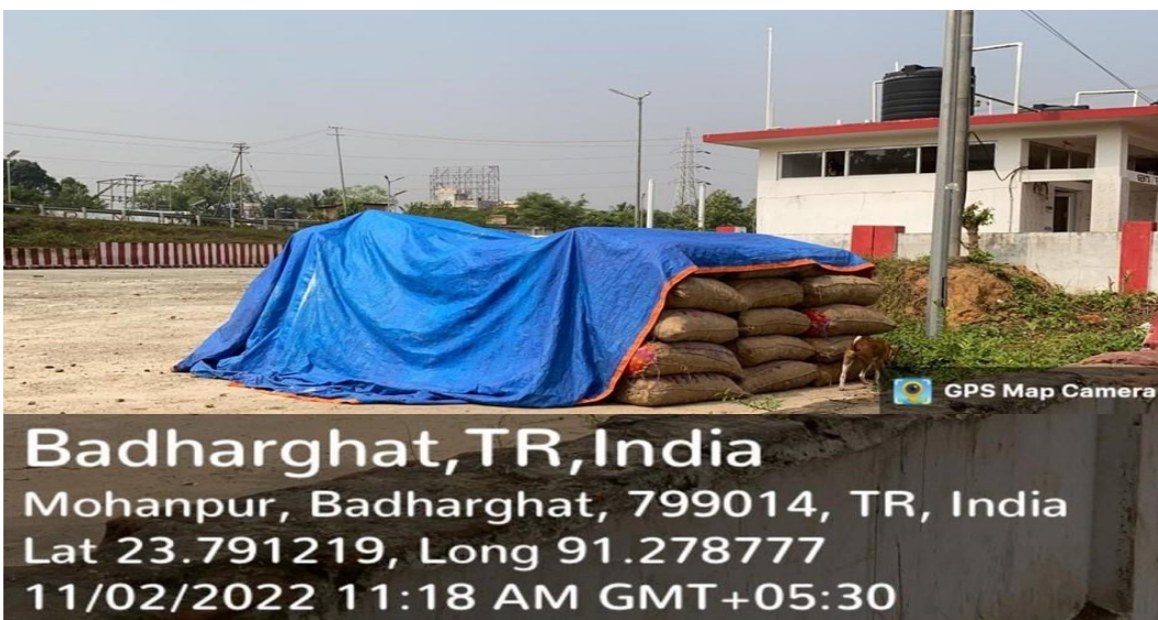
Agartala Station of Northeast Frontier Railway
