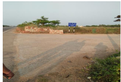
Photo No.32: Completed portion of road - Khandia Bandha to NH by-pass (NH-316)
