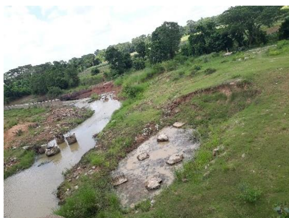
Photo No.28 - Bridge at chainage 11.050 km
