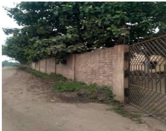
Photo No.10: Boundary Wall of Thelkoli HS
