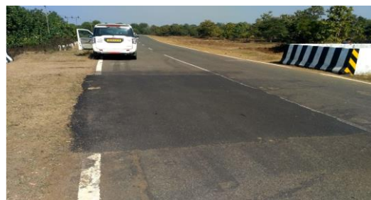
Photo No. 15: Patch work at RD 137.64 km of Ghatipada - Ampani road
