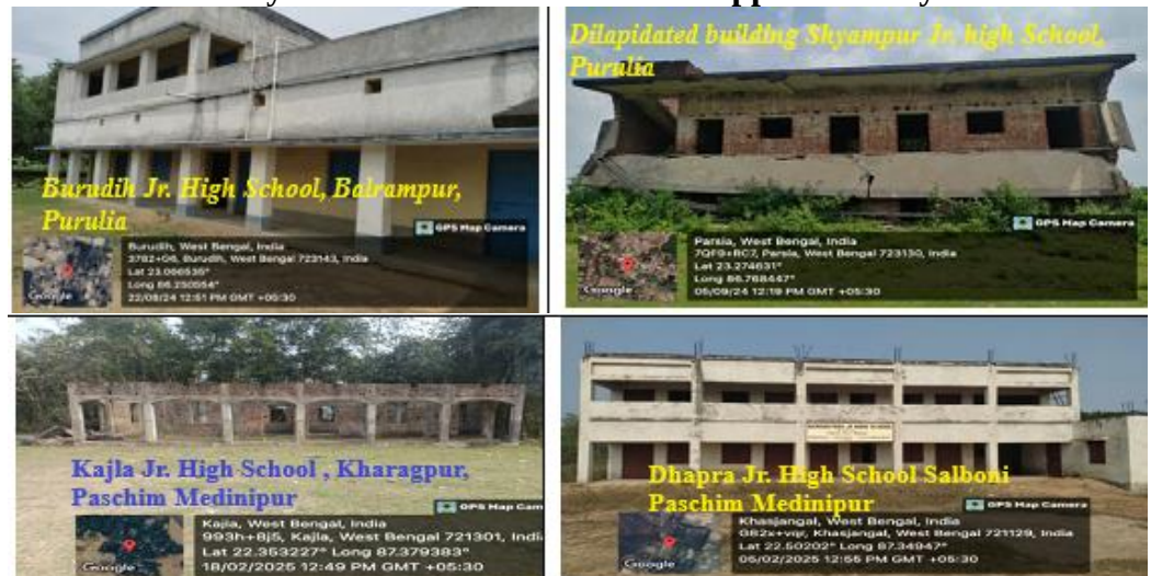
Picture 6.5: Newly constructed non-functional Upper Primary schools
