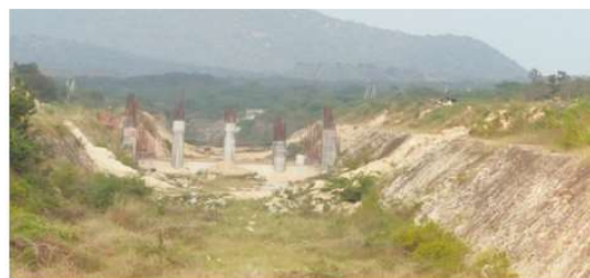
Incomplete structure on Feeder canal
