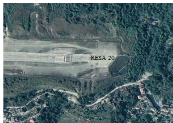
Figure 1.8: Runway End Safety Area at RWY20
