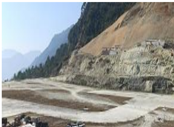
Figure 1.4: Ongoing work of concrete cladding wall
