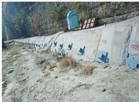
Figure 1.5: Ongoing work of strengthening the base of the retaining wall
