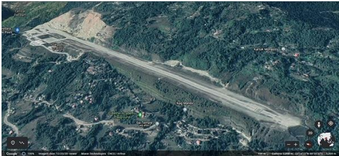
Figure 1.6: Runway at Pakyong airport, Sikkim
