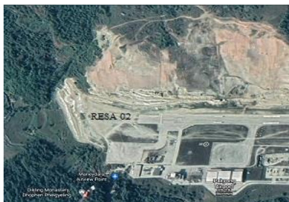
Figure 1.7: Runway End Safety Area at RWY02
