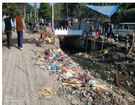
Fig.2.18: Garbage dumped at roadside at Shantinagar, raised pedestrian walkway, parallel road under Alipurduar PW Division (20.12.2020)
