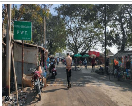
Fig.2.16: Encroachment of shoulder of Cross road by shops near Radhamadhav Mandir and Kaljani Housing complex under Alipurduar PW Division (20.12.2020)
