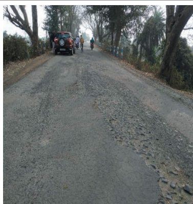
Fig.2.4: WMM exposed at 9.5 km of Simlipal-Sarenga- Bamundiaghat Road (16.01.2021)
