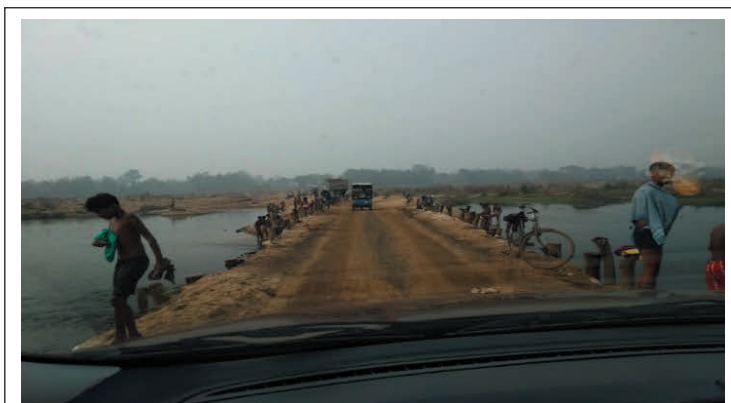
Fig. 2.12: Chandrakona-Goaltore-Sarenga-Simlighat Road of Bankura Highway Division. A make shift bridge which becomes unusable in monsoon
