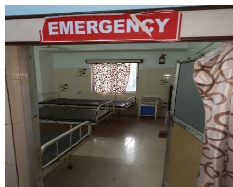
Picture 1.4: No facilities available, only beds kept in an area earmarked as an emergency ward (Loknath Nursing Home, Birbhum).
