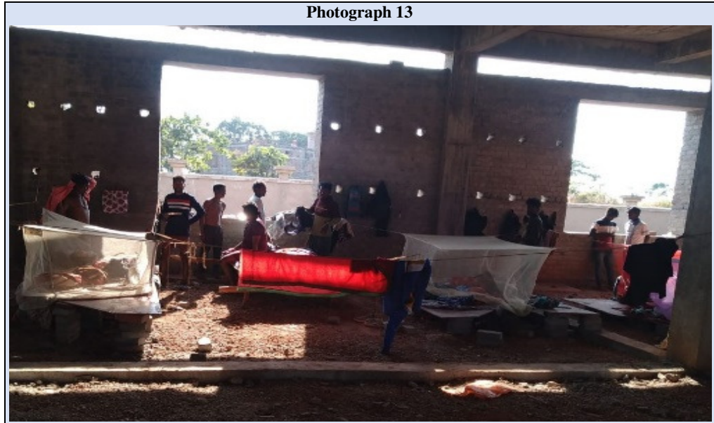
Workers residing in an under-construction building, at the construction site of the PM Awas Yojana, at Birsa Nagar, East Singhbhum (23 November 2022)
