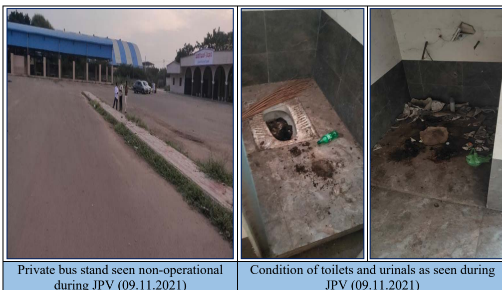
Exhibit 3.2: Status of private bus terminal constructed at Ballari
