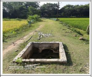
Photograph 3.3.4:Inspection chamber of sludge disposal remained incomplete
