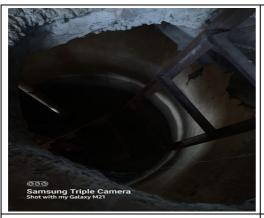
Photograph 3.3.1: Bottom floor of intake well remained incomplete
