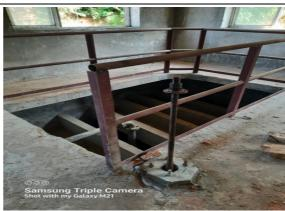
Photograph 3.3.2: Operating System of Sluice Valve remained incomplete
