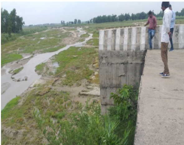
Picture No. 3: 16x25 bridge at chainage 67.21 (river)
