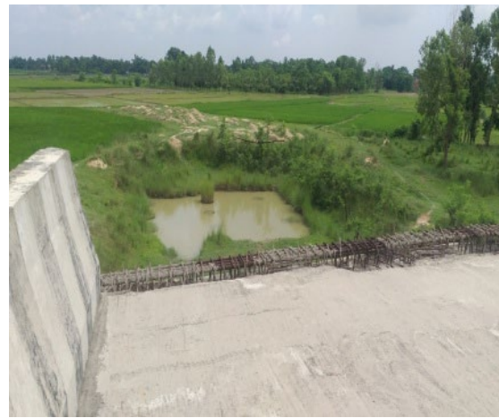
Picture No. 4: 7x30 bridge at chainage 75.734 (agricultural land)
