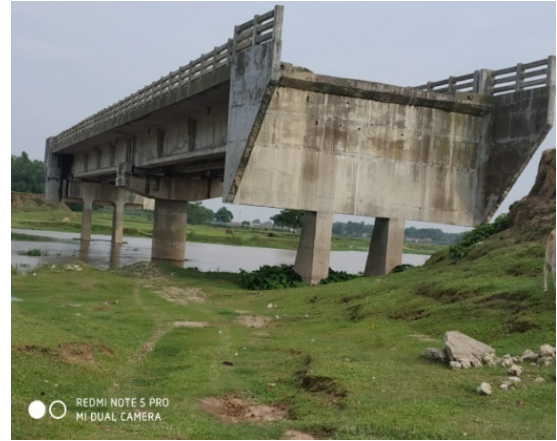
Picture No. 2: Jobna river (chainage 123.30) in Kishanganj district
