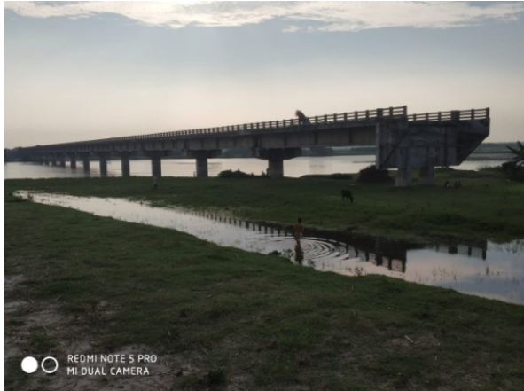
Picture No. 1: Galgalia to Pintola in Kishanganj district under Mechririver (chainage 124.12).
