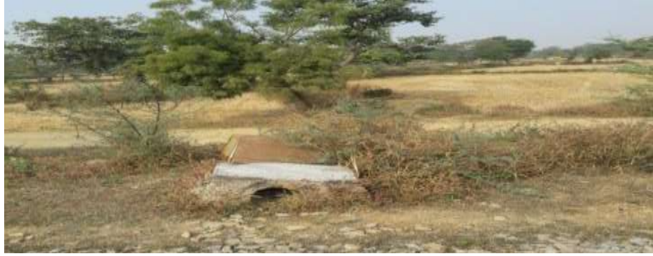
Steel apparatus case of automatic signalling system lying demolished at railway line between stretch of Bridge no.17 and null point of cutting section.
