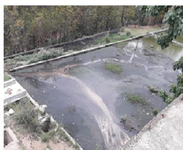
Uncovered sludge drying beds inundated/ overflowing with water at STP, Shanti, Solan (05 June 2018)
