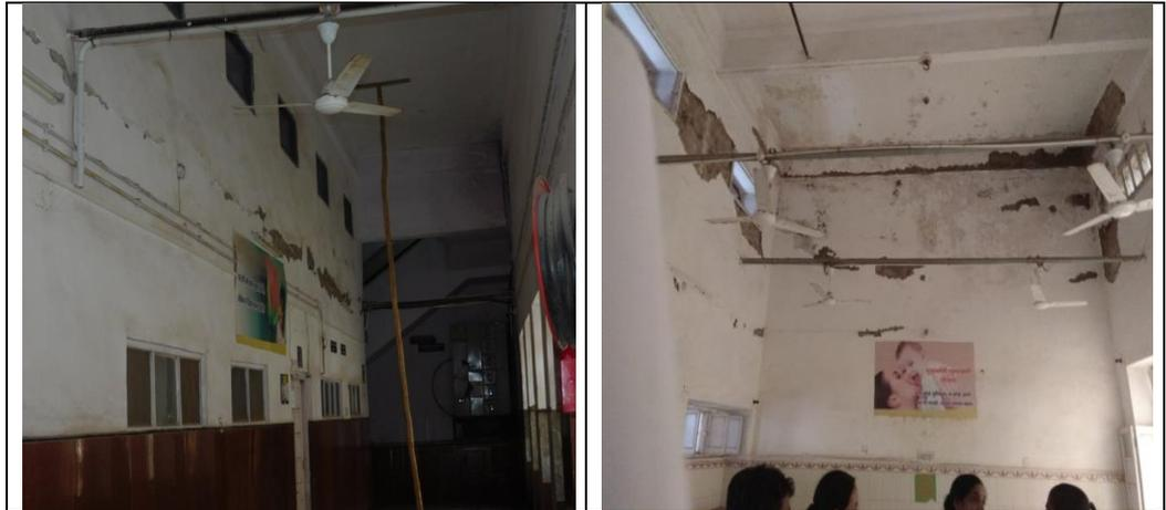
Horizontal cracks in the walls, lintels and roof of Government Pannadhaya Hospital, Udaipur
