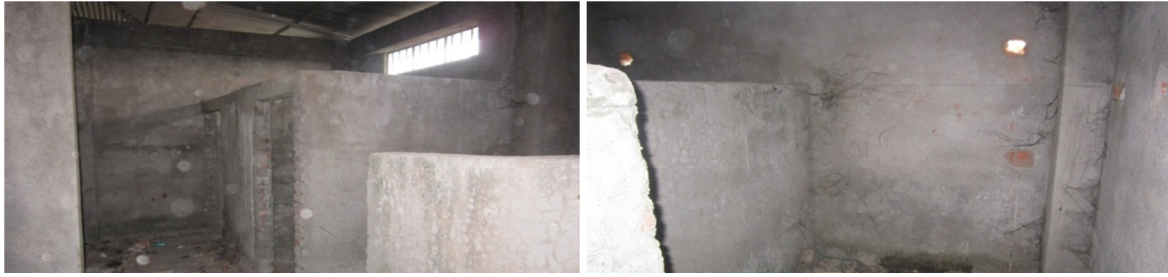
Photographs of Business Center in Dokmoka Town, showing no evidence of any service works being done
