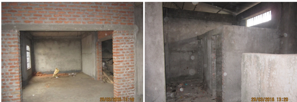
Photographs showing incomplete state of work of the Business Center at Dokmoka Town
