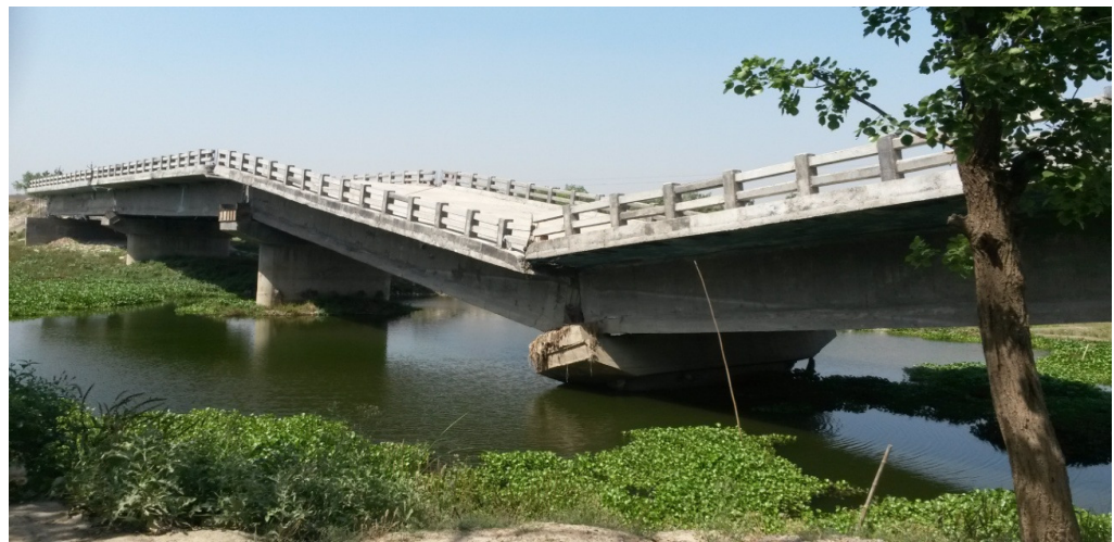
Damaged bridge on Runnisaipur-Katra-Kewatsa Road in Muzaffarpur
