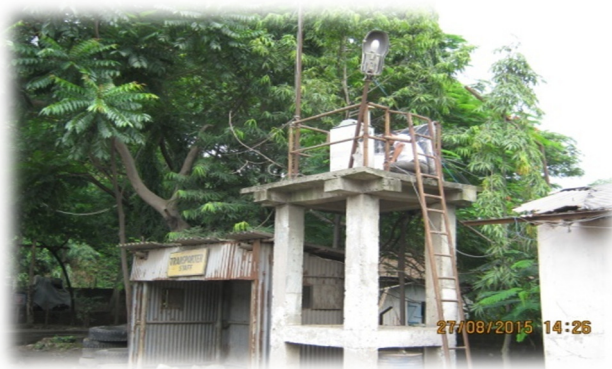
Air Monitoring station at premises of M/s Purbanchal Cement
