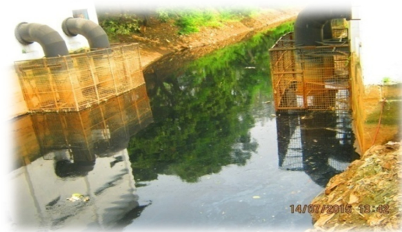
Drainage outlet at Bharalumukh
