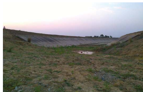
Collapsed portion of SMC from RD 7950 to 8720 M
