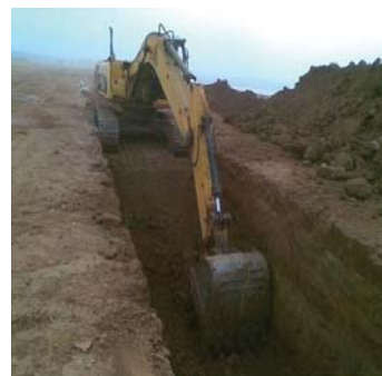
Excavation of vertical chimney by mechanical means
