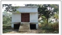
Photograph of RPWS at Janged in Bargarh district which remained non functional due to non completion of electrification works
