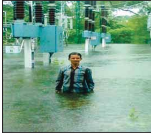
File photo of 132KV SS Bhopatwala Haridwar during flood
