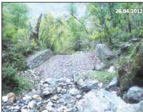
Check Dam Nirman, Year 2009-10 Quarijimiya GP, Munsyari Block, District Pithoragarh
