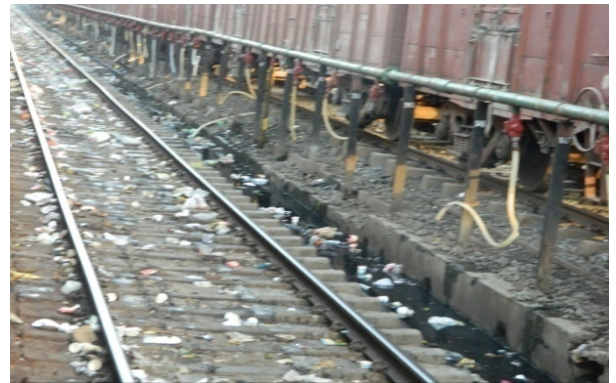
Drain along side the track clogged with garbage (Bilaspur/ SECR)
