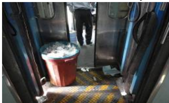
Vestibules used for storing garbage
