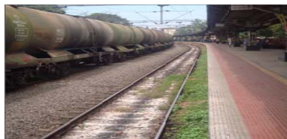
Human wastes in track covered with lime/bleaching powder at Ernakulam Town, SR
