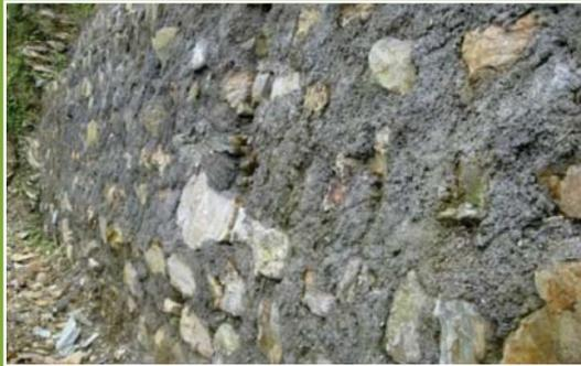
*Protective walls constructed under PMGSY by the Department with random size of stones, non-use of appropriate bond stones and weep holes*
