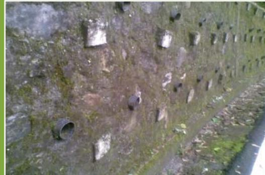
*Sample protective wall constructed with appropriate use of bond stones and weep holes*
