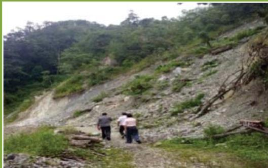
Rampant land slips due to hill cutting
