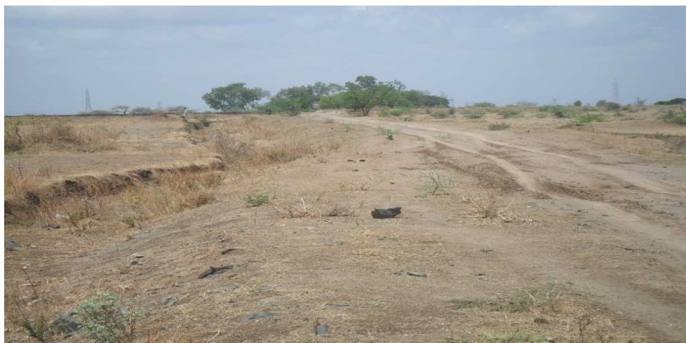
Photograph of incomplete road work at Bangla Tanda; Taluka Paithan; District Aurangabad
