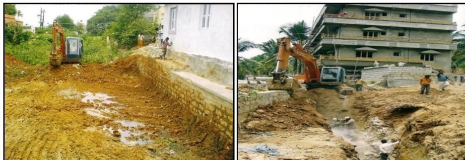
Earthwork excavation by mechanical means in Vrishabhavathi valley
