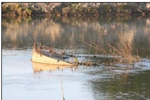
**SHIFT AND TILT OF SUBMERGED PIER NO.1 (26/12/2011)**
