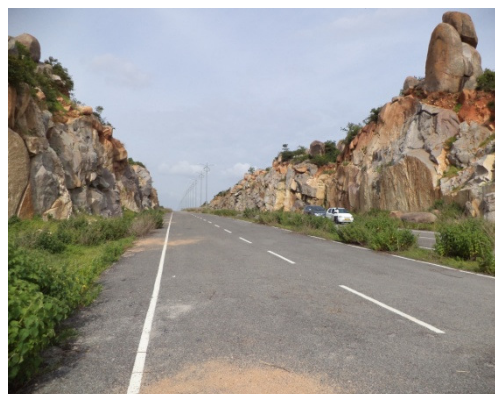
Road aligned through hard rock hillock
