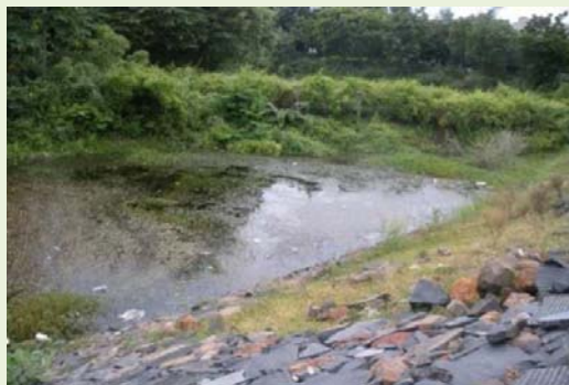
View inside Lakaram SS Tank
