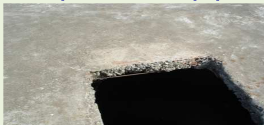
Sump without water vents
