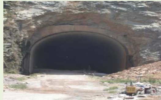
Tunnel work at Gandikota Reservoir under progress
