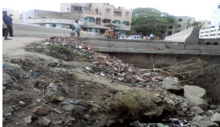
Figure 1 : Bridge near Gun point
