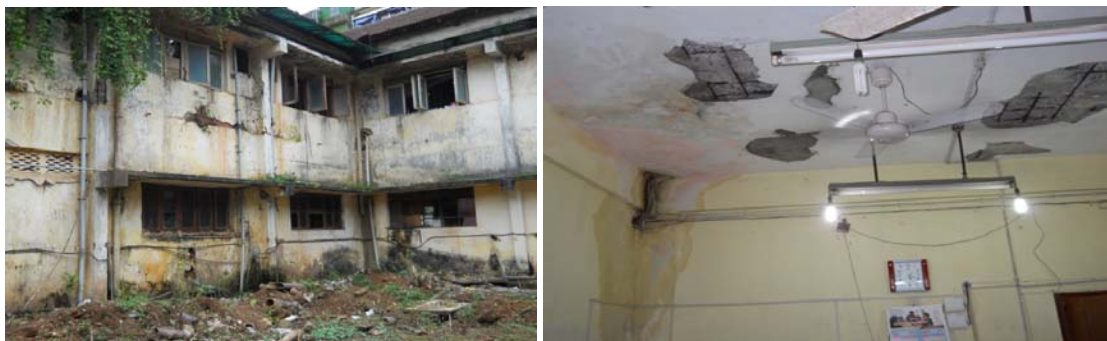
External and internal view of old Asilo Hospital
