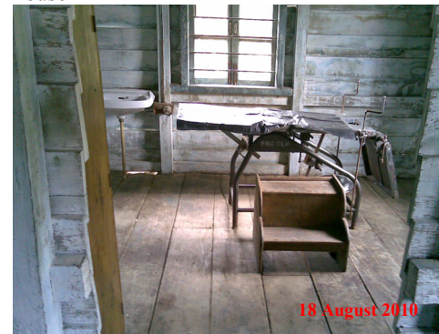
Poor state of Labour Room at PHC Thanlon, Churachandpur
