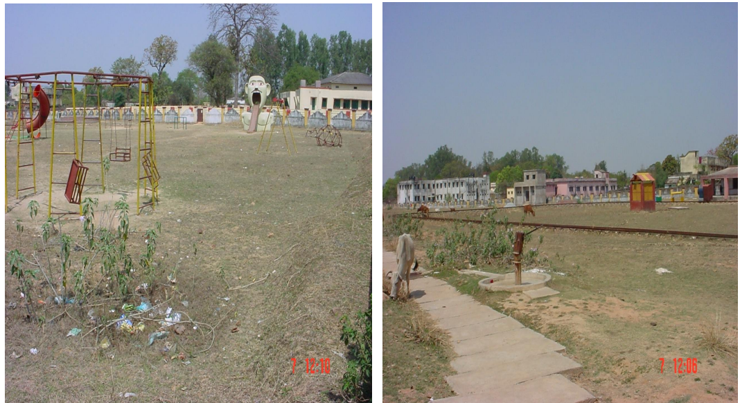
(Photos showing incomplete/damaged work of construction/beautification of Park at Simdega)
