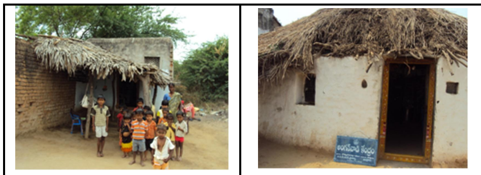
AWCs functioning ( 13 th & 20 th March 2010) under a small roof in Udatalapalli (V) (Nalgonda District) and dilapidated kutcha house in Bommarajupalli (V) (Guntur District)
