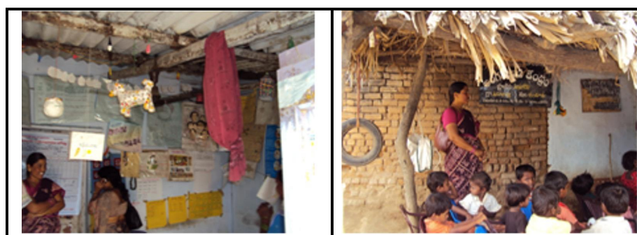
AWCs functioning (20 th & 13 th March 2010) without basic infrastructure facilities in Ipur (V) (Guntur District) and Udatalapalli (V) (Nalgonda District)
