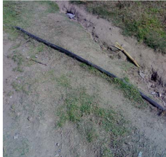
Picture: 3.1.14 Open pipeline
