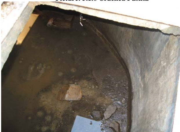
Picture: 3.1.7 Supply Tank
