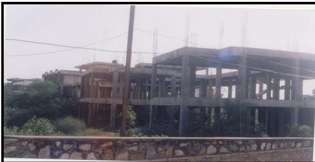
A view of incomplete staff quarters
