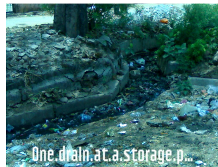
One drain at a storage point in Rourkela Municipality blocked due to plastic waste
