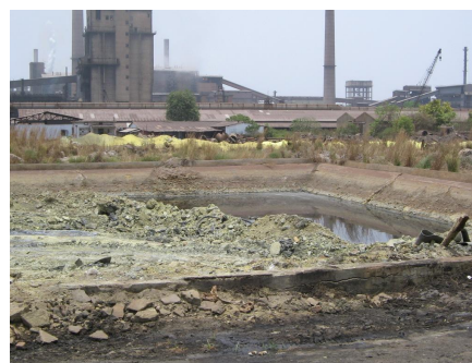
Hazardous waste pit 1 partly filled with water at RSP dated 7 May 2008
