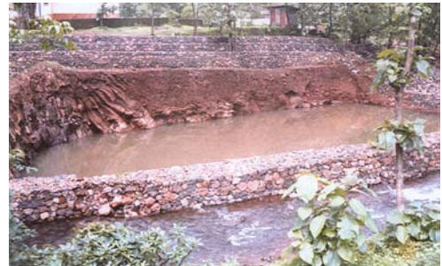
Water tank at Lanja, District Ratnagiri showing muddy water unfit for drinking.
