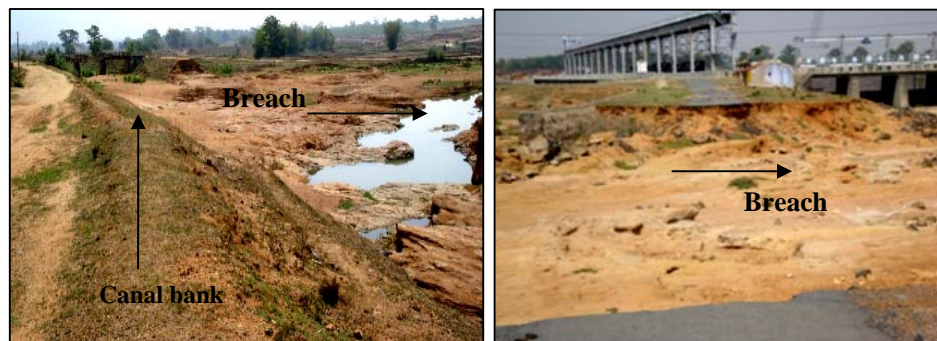
Photographs taken on 29.5.2008 showing damaged main canal and approach road to barrage in Sikatia premises near the barrage had been abandoned by the officials.
