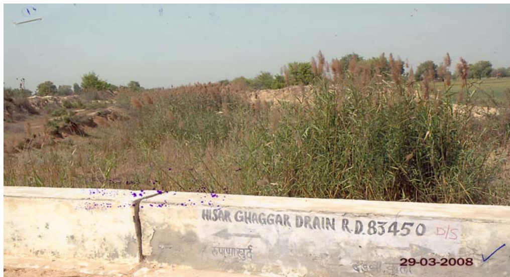
Non-functional Hisar Ghaggar drain at RD 83450
