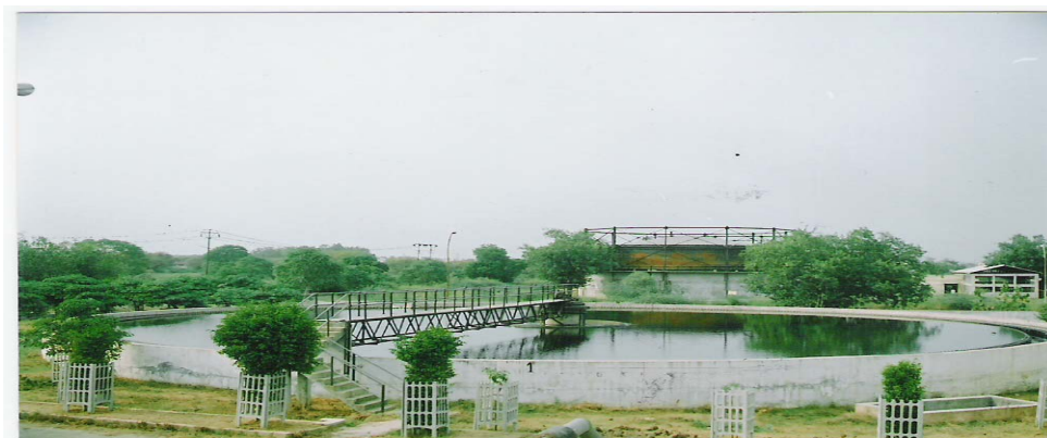
Figure-12: A view of the gas chamber and sewage settling plant
