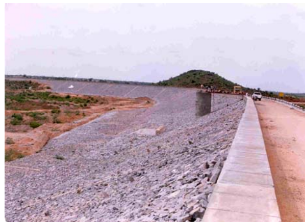
Cistern earth dam at Paluguthanda (v), PA Pally (M) (Nalgonda District)
