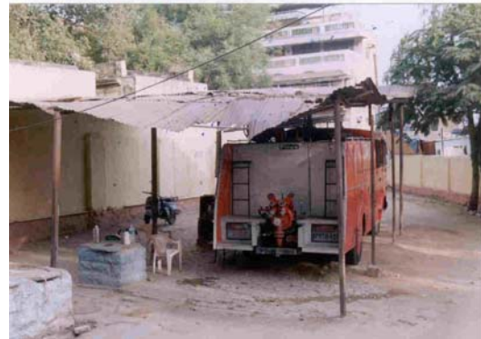
Fire Station in temporary structure, Gowliguda, Hyderabad
